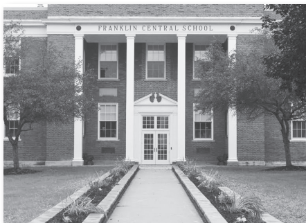
NEW FLOWER BEDS WERE INSTALLED ON THE FRONT WALKWAY
