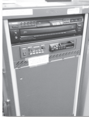
Replace PA system
