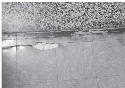
Replace worn and damaged floor tile & carpet
