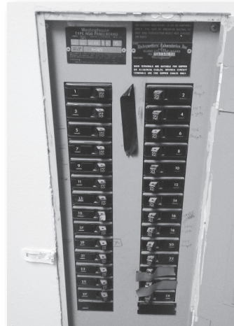
Upgrade electrical system
