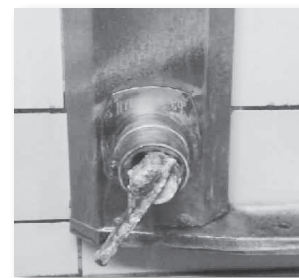
Replace broken shower valves
